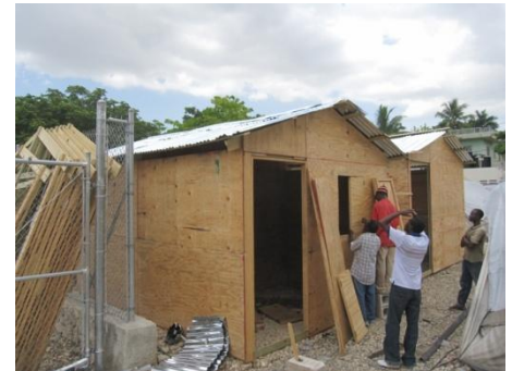
Completed transitional shelters in downtown Port-au-Prince.
